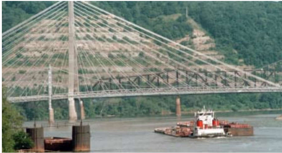
The Veteran's Memorial Bridge is the county's link to Pittsburgh.
